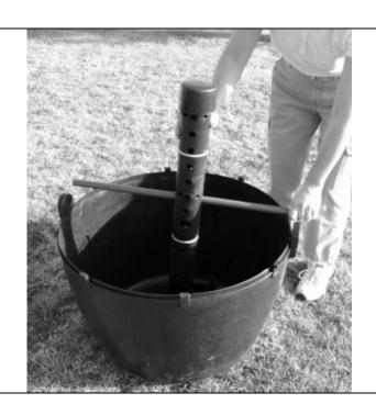
Check and be sure the aeration tube has been snapped together, secured with two Ty-Wraps, the cap is snugged down and the breaker bar inserted.
